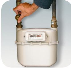
Get into the habit of turning off the gas at the meter, or on the pipe coming into your home, when you are not using gas-burning appliances. Always do this when you go away, even if you will only be away for a short time.
